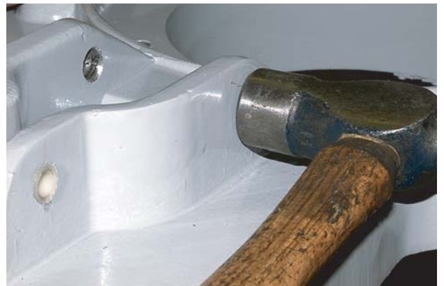
4. Hammer bushing in, flush.
